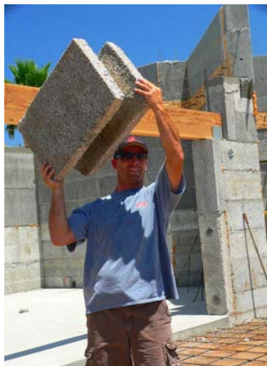
Valade hoists light-weight and fire-safe Perform Wall block
