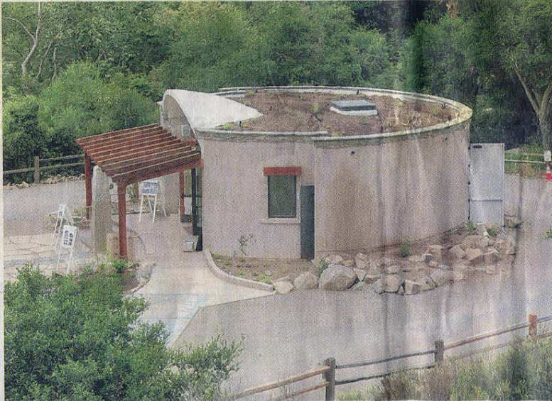
The center is shown as it neared completion in early May. Set in a canyon amid the natural habitat of Elfin Forest, the center will provide educational information. Charlie Neuman | Union-Tribune
